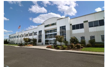
Barnes & Noble Distribution Center Monroe, NJ
