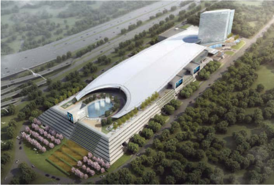
THE MGM NATIONAL HARBOR RESORT IS SET ON A PEDESTAL, EVOKING A MONUMENT AND INCORPORATING A SEVEN-STORY PARKING GARAGE. A SKYLIGHT RUNS THE LENGTH OF THE ROOF BETWEEN THE OUTDOOR TERRACE AND HOTEL TOWER.
